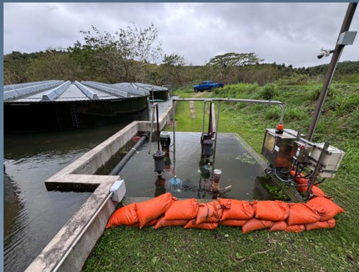
Leachate Tanks/Pumps on 4/16
